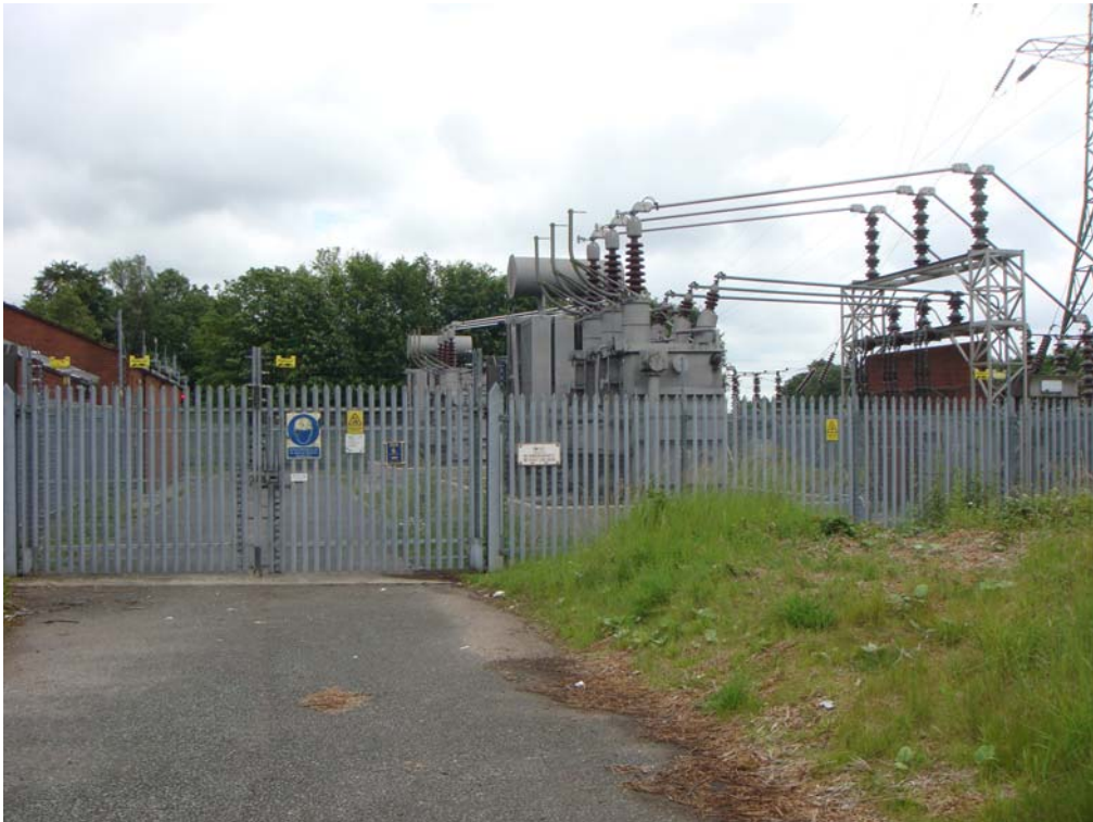
Photograph 1 – General view from the access road
