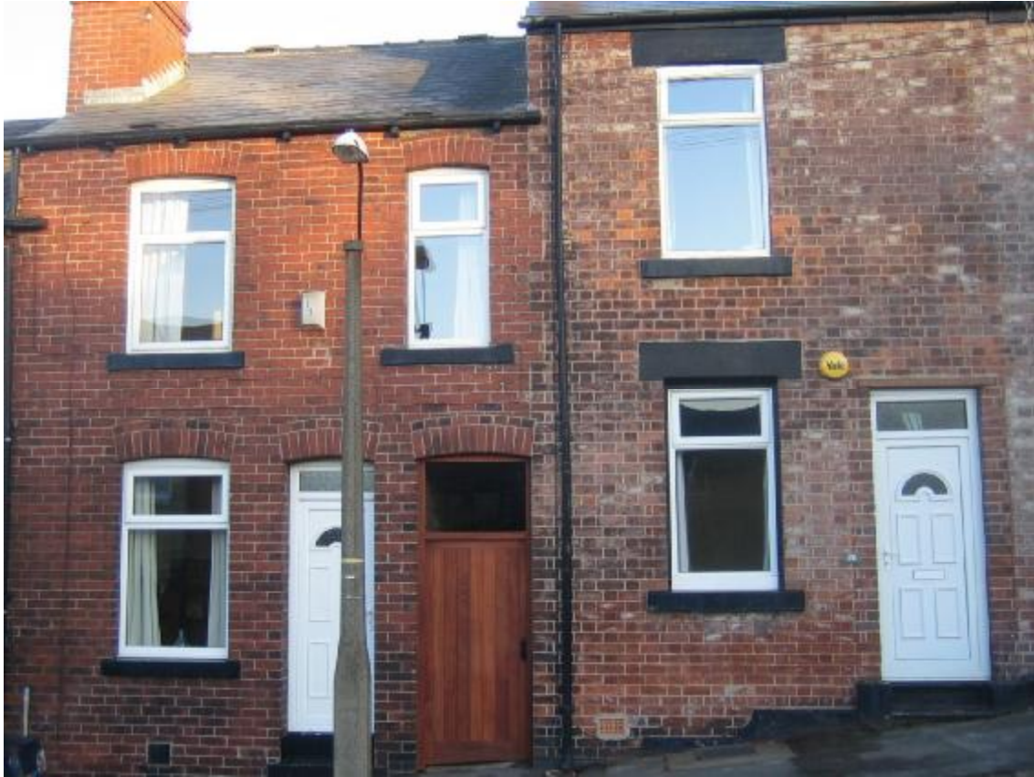
Figure 1 – Custom built walk-through door fitted with single glazed toughened glass panel above
