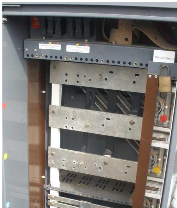
Stripped out interior of LV transformer mounted cabinet illustrating horizontal, forward facing and diagonal main copper connections, normally hidden behind shrouding and fuse carriers. This copper work is live in service at 400 – 415 volts and rated for a short circuit level of 50,000 amps.
