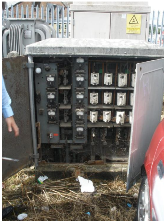
Old style outdoor LV fuse pillar. Fuse carriers are in place, but the older designs do not have the safety shrouding of modern designs
