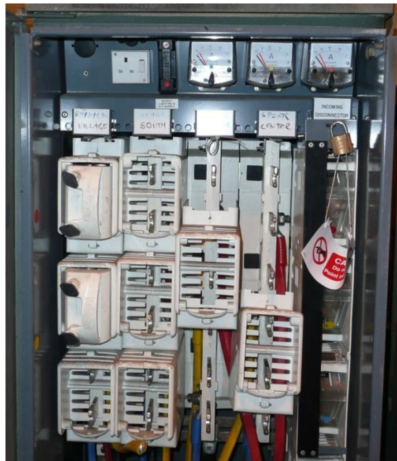
Modern LV transformer mounted LV fuse cabinet – in this photo two fuse carriers are in place. Under normal circumstances all LV fuse carriers would be in situ.
