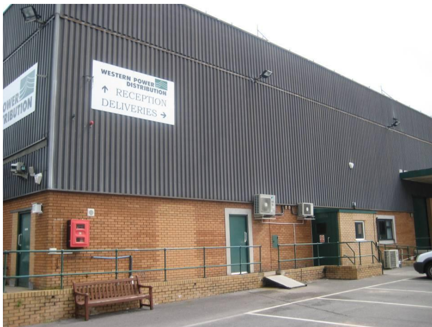
10.31 The ground floor area was mainly given over to a new, high density centralised storage facility.
