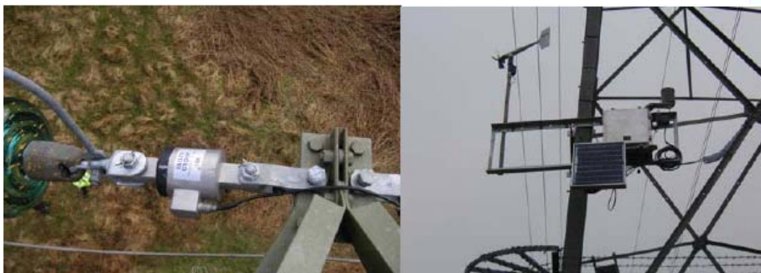
Typical CAT-1 Installation on SHETL Transmission Circuit
