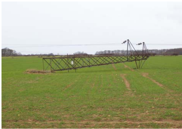
Figure 1 – A Failed 33kV Steel Tower - The result of high corrosion levels and a high mean wind speed!
