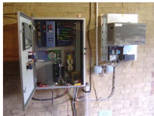
Figure 5 The 4Energy Midi BAC (right) with a London distribution substation Remsdaq RTU
