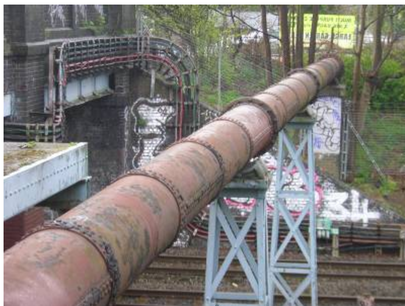
Figure 3.23 - Sheepcote Road Rail and Underground Crossing
