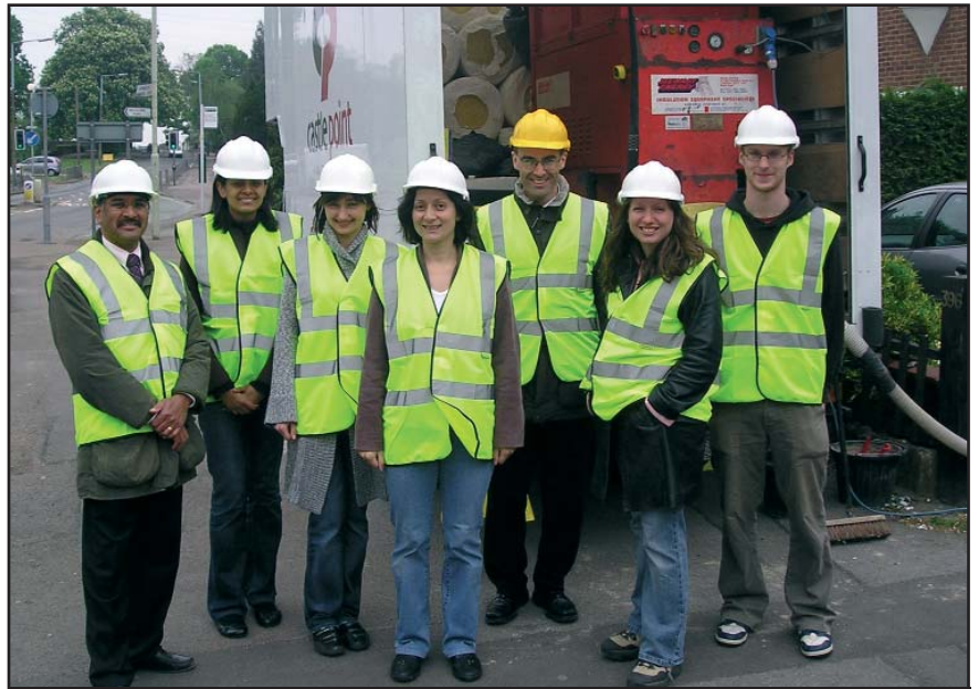
The Ofgem Energy Efficiency team visited a home to watch insulation being installed. From left to right : Dinesh Naidu, Priya Patel, Urszula Kulpinska, Sue Corbett, Charles Hargreaves, Emily Flatt and James Clee.
