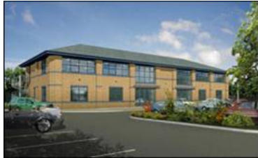
Hedon, near Hull Administration/engineering
