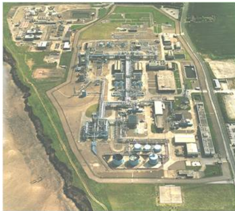
Easington Terminal Rough gas processing Amethyst gas processing Tie in to National Transmission System 24/7 Operation
