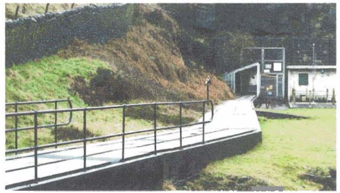
Surface troughing crossing the river Etherow and entering the Woodhead tunnels (carrying six 400kV cables - a double circuit)
