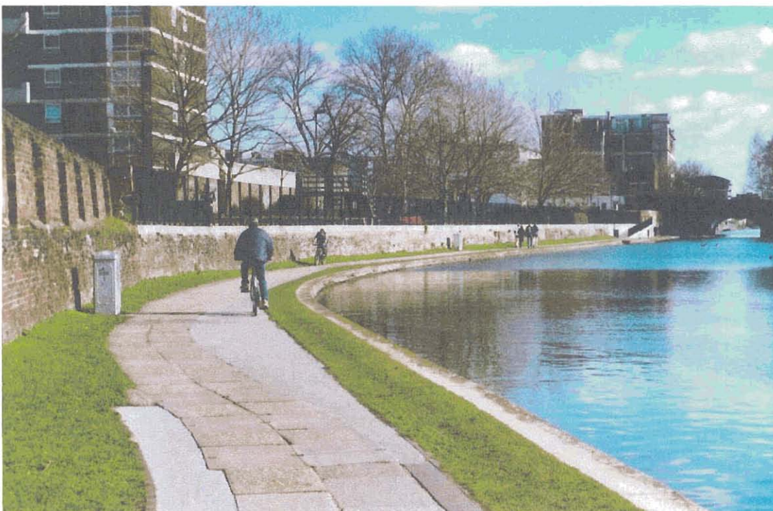
Pedestrian route above six 'undergrounded' NG 400kV cables in Regents Canal towpath, London.
