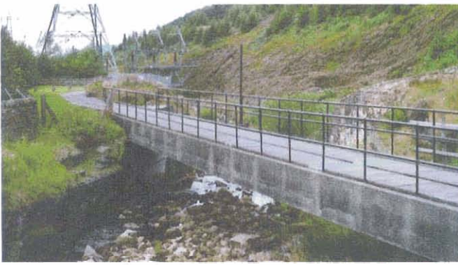
Surface troughing crossing the river Etherow and entering the Woodhead tunnels (carrying six 400kV cables - a double circuit)
