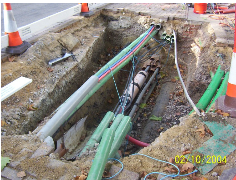
Image 1: Shows the extensive size of excavation in footways often required to identify LV cables amongst those of other services (British Telecom in grey and other telecoms operators in green). All require careful hand excavation to avoid damage. Excavation close to the roadway constrains working space.
