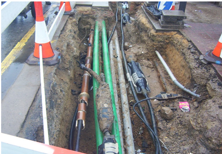
Image 1: Shows the extensive size of excavation in footways often required to identify LV cables amongst those of other services (British Telecom in grey and other telecoms operators in green). All require careful hand excavation to avoid damage. Excavation close to the roadway constrains working space.
