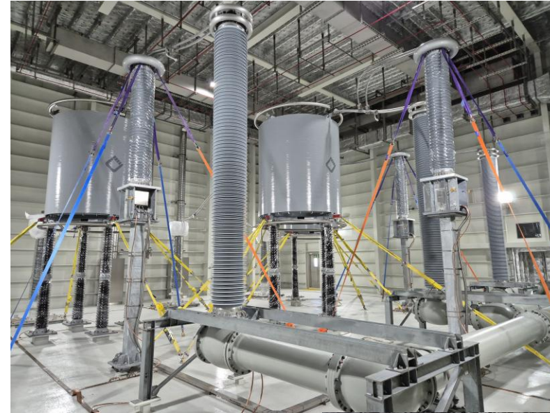
Reactors with sea-fastening in place (right)
