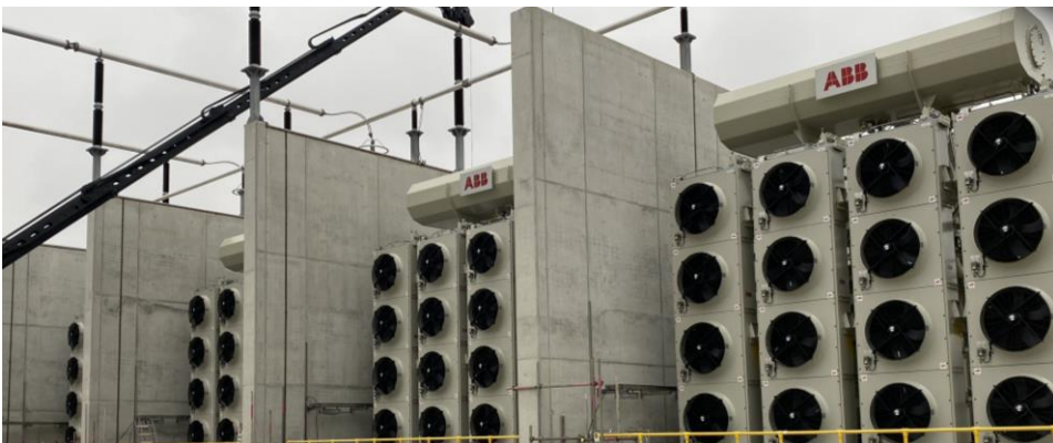
Converter Transformer Units
