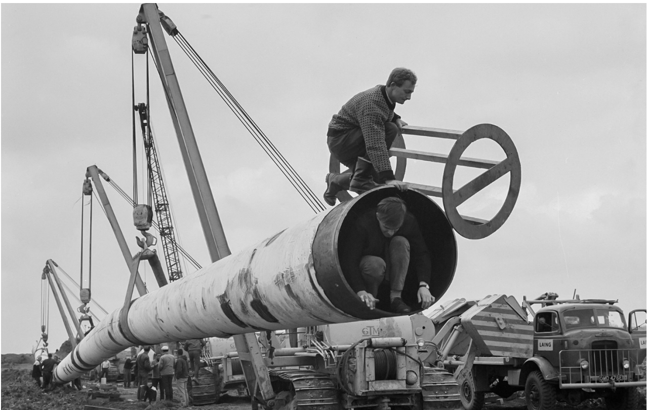
Image: The Fens gas pipeline being lifted by a row of Caterpillar 583 pipelayers. Work on laying the Fens gas pipeline started in June 1967. Over 600 men worked on the project to lay 36 inch diameter steel pipes which crossed four rivers and numerous dykes and ditches. (Heritage Image Partnership Ltd / Alamy Stock Photo)
