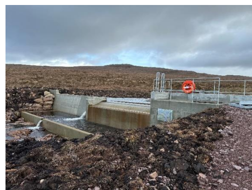
Figure 2 – intake to penstock from Reservoir
