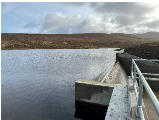
Figure 2 – intake to penstock from Reservoir
