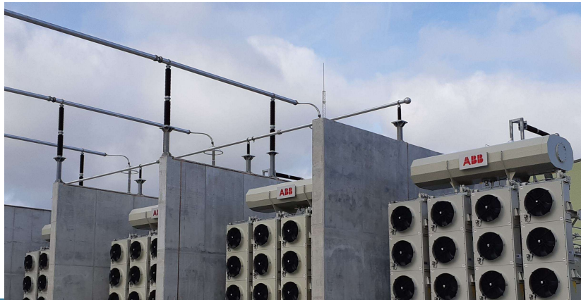
Single-phase Transformers (L)
