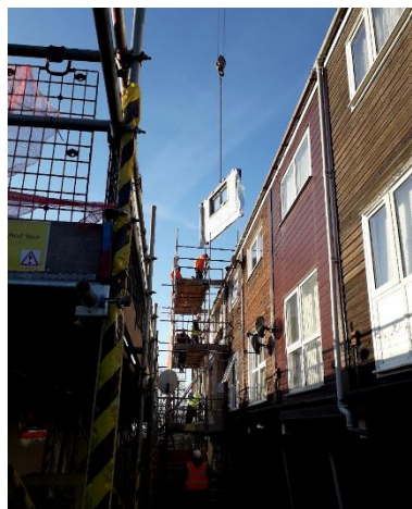
During panel install
