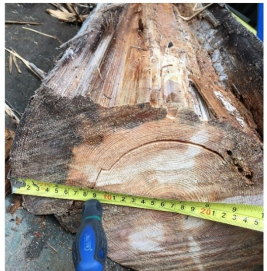
Wood pole decay
