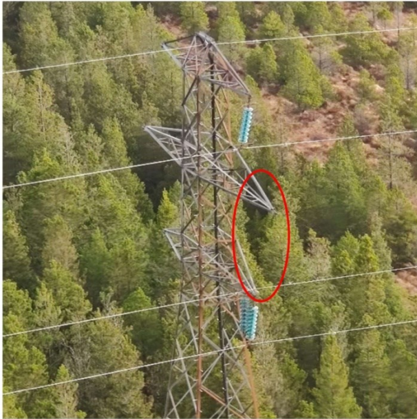
Middle phase shackle failure
