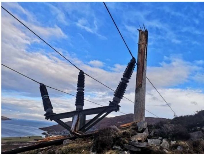
Wood pole failure
