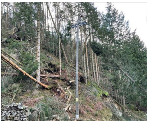
Figure 4 - 33kV pole bending under weight of fallen tree on conductors (Comrie, Perth and Kinross)
