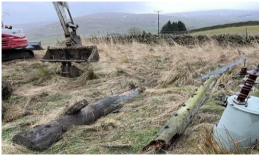
Figure 6 - Pole damage from suspected line icing (Weardale, County Durham)
