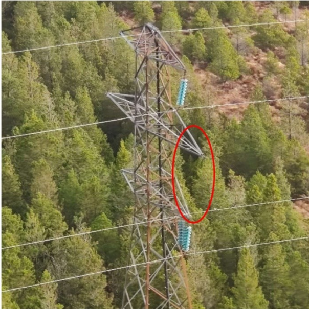
Middle phase shackle failure
