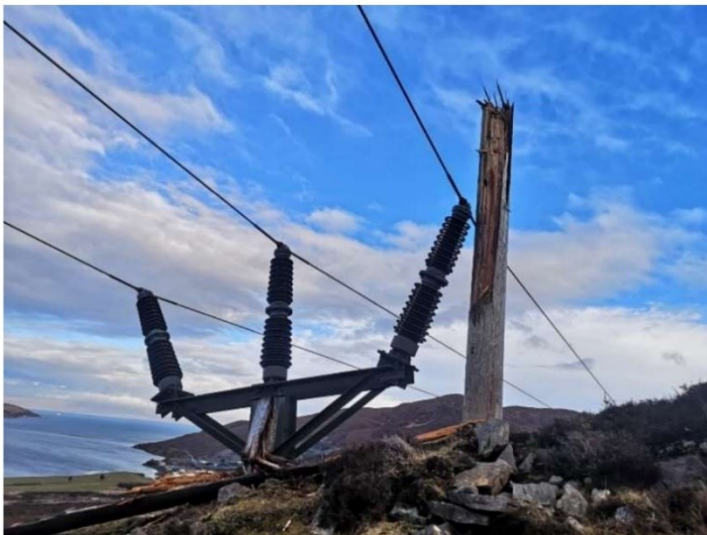
Wood pole failure
