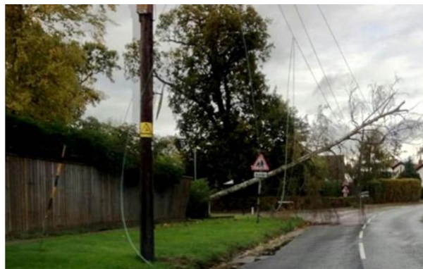
Figure 6 Tree suspended by open-wire LV overhead line
