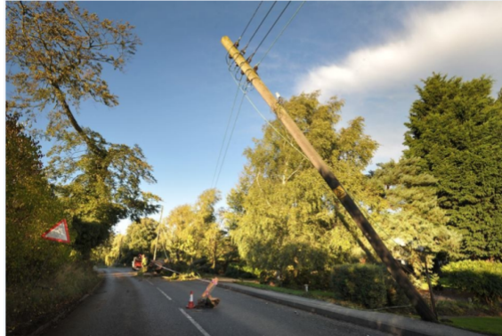
Figure 5 Tree through overhead line
