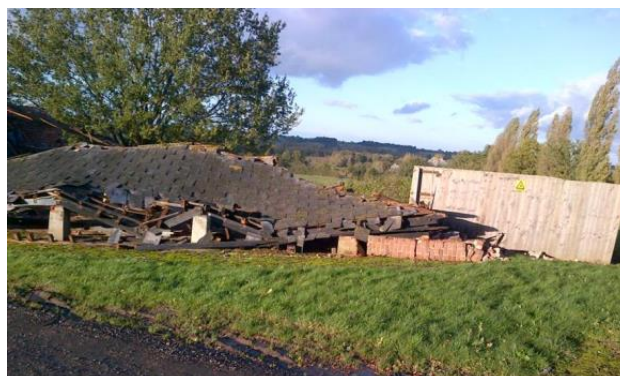
Figure 3 Building collapse onto adjacent substation
