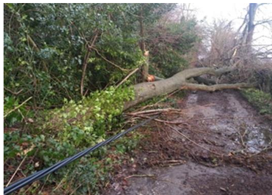
Figure 7 Tree brought down an ABC LV overhead line
