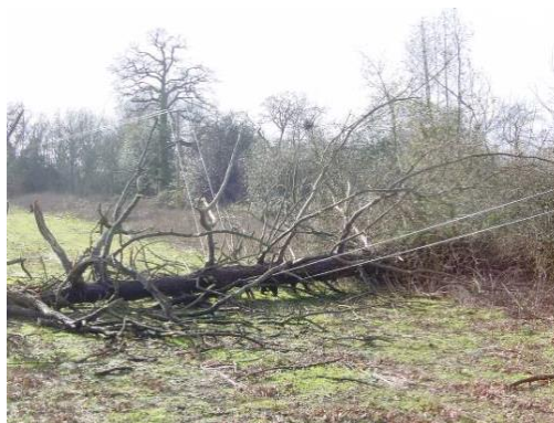
Figure 8 Tree brought down an HV overhead line
