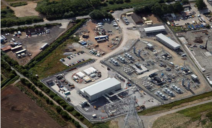
Onshore Substation (Q3 2013)
