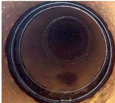
Figure 2 - Weco Seal Installed In Pipe
