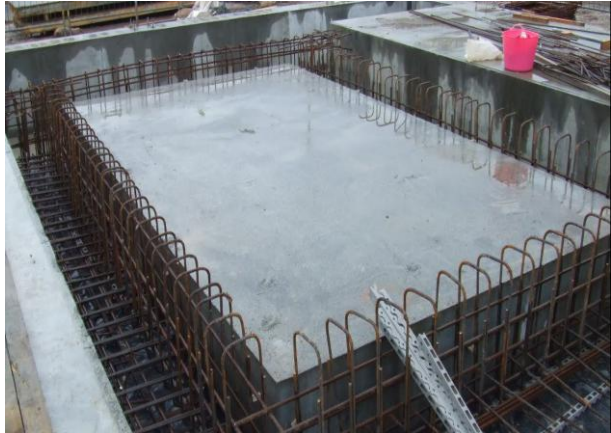
March – Concrete and rebar laid, foundations complete
