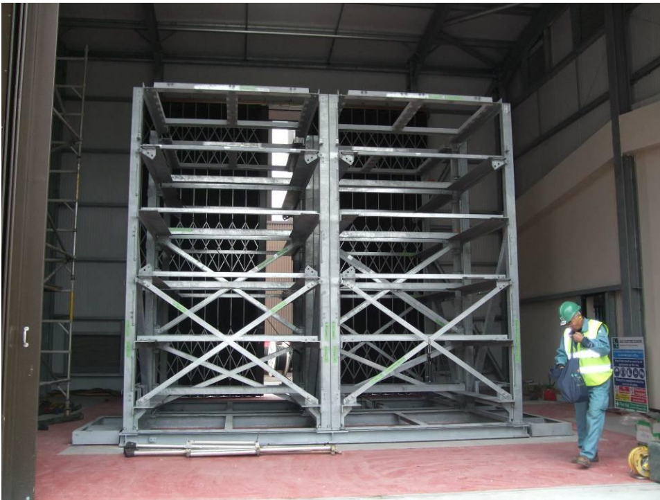
Figure 11 - Installed battery enclosure frame
