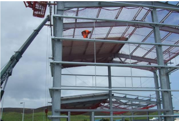
April – External building frame erected
