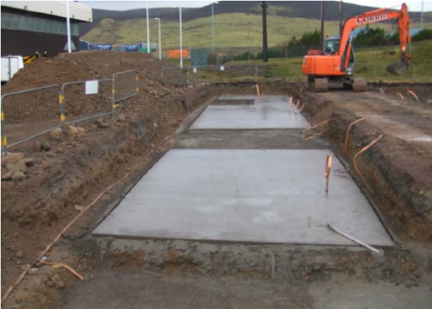
February – CDM site initiated, site excavation, first concrete poured
