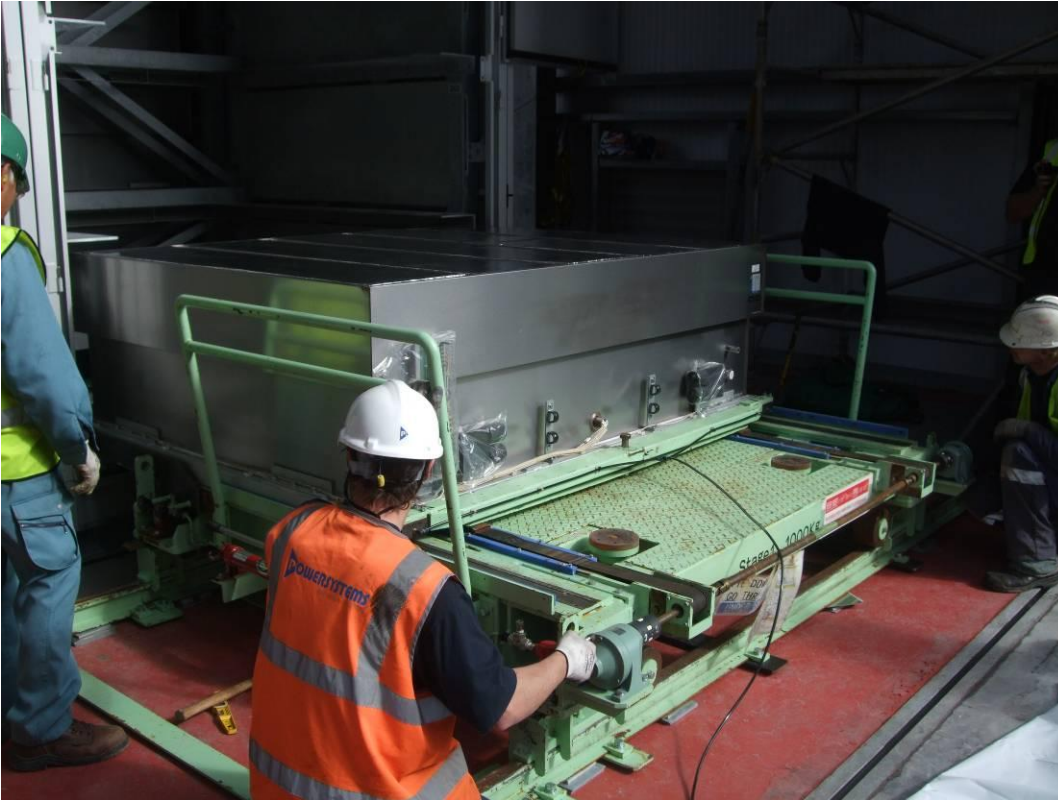
Figure 13 - Battery module insertion
