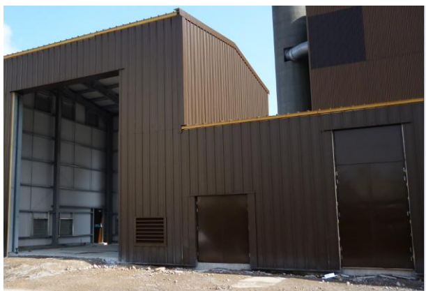
May – Building fully clad, internal works begin
