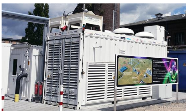
Figure C.3.1 ITM Power's Grid Connected Electrolyser in Frankfurt, Germany
