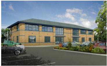
Hedon, near Hull Administration/engineering
