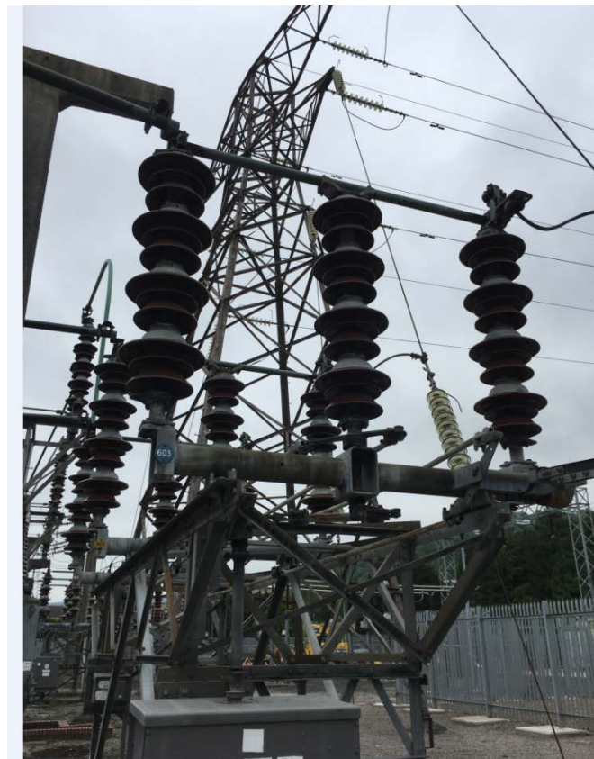
Figure 2: 132kV RCP Disconnector at Galashiels 132kV substation
