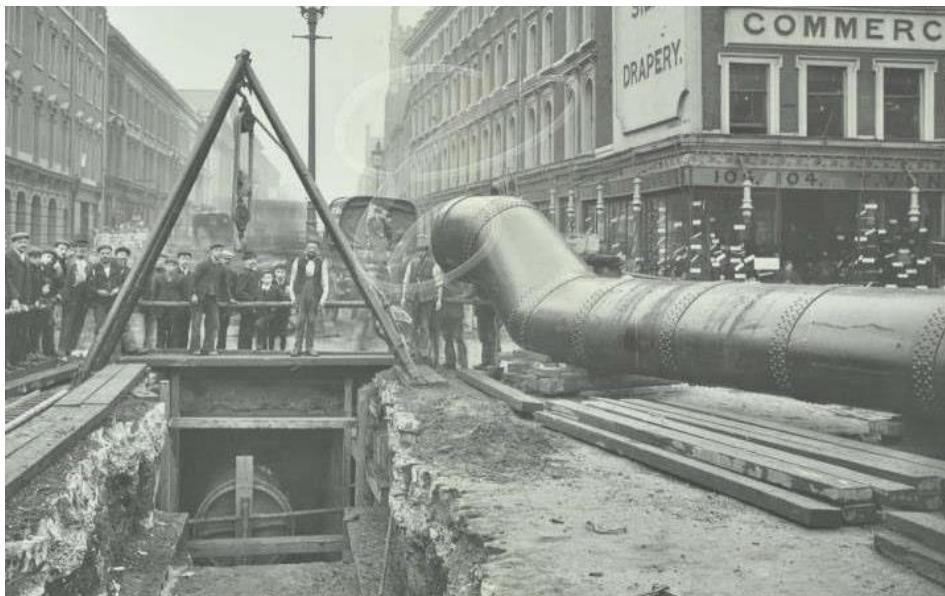
Figure 1: 48" Iron Elliptical main at Commercial Road c. 1906
