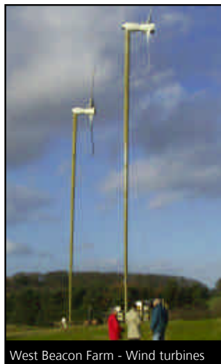
West Beacon Farm - Wind turbines
